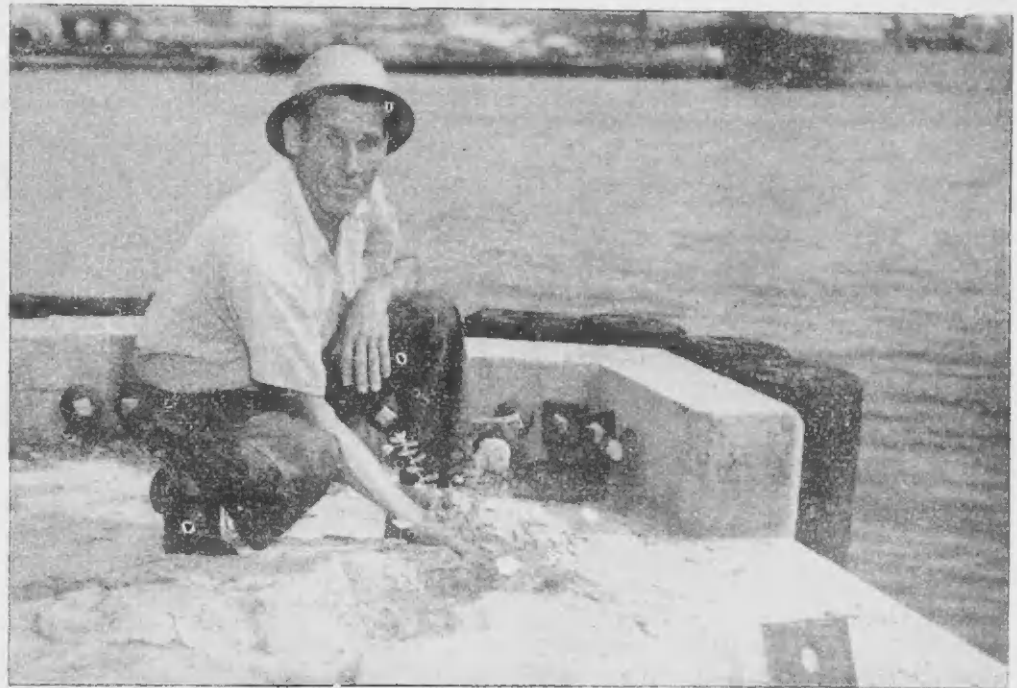
Probably the hardest and loneliest of all flowers in Aruba are these wild "buttercups". They are growing out of a few handfuls of sand that the contractors left on top of a 40-ton block of concrete that perches on some steel piles in the harbor. Aruba's sand and sun can be very nourishing — especially if no one cares whether the plants grow or not. Holding up the flowers is Wharfinger Adrian Geerman, who has been keeping track of things around the harbor for 24 years.
